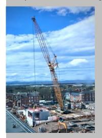
Pre-formed concrete sections of the structure are being assembled on site with the help of a large mobile crane.
