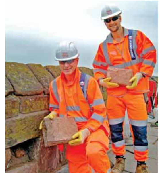
Two generations of local stonemasons, father and son, Martin and Jack Rigby working on the city walls in Nun's Road, using Roman stone blocks recovered from the Northgate site
